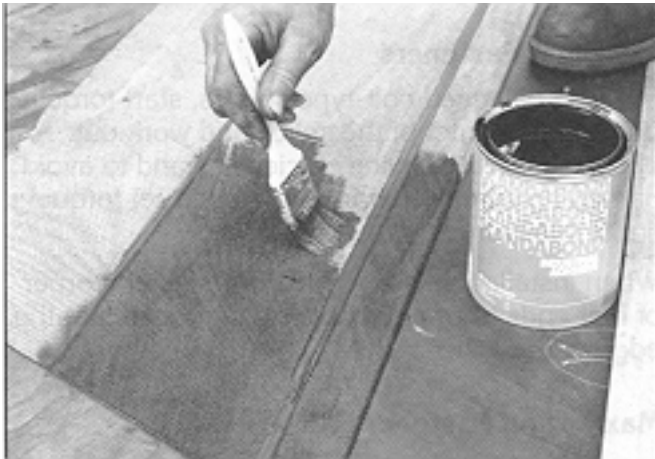
Figure 5 Use only the best grade of splicing compounds such as Scandabond adhesive.
