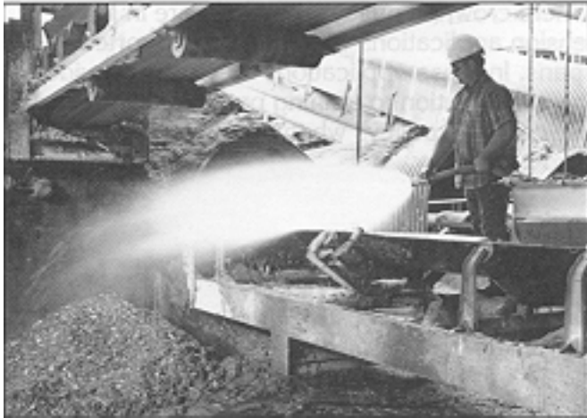
Figure 8 Hosing away spilled material.
